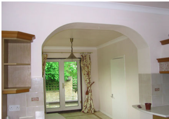
Existing kitchen, with false arch
