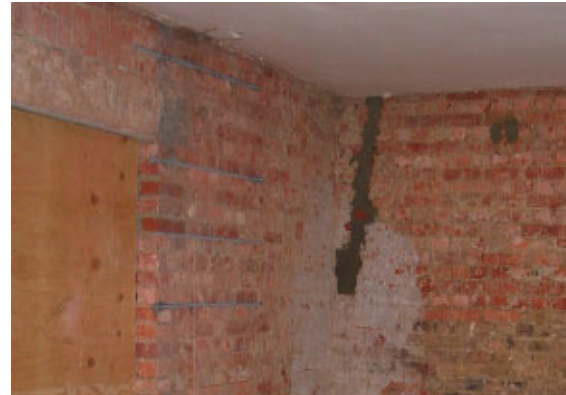
Brickwork repair internally (Helix bars)
