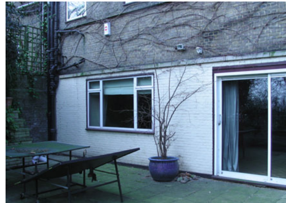
Rear elevation prior to cleaning and paint stripping
