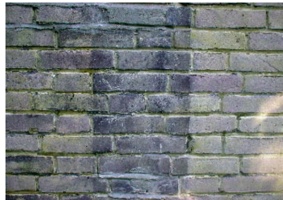
Tests of cleaning carried out
