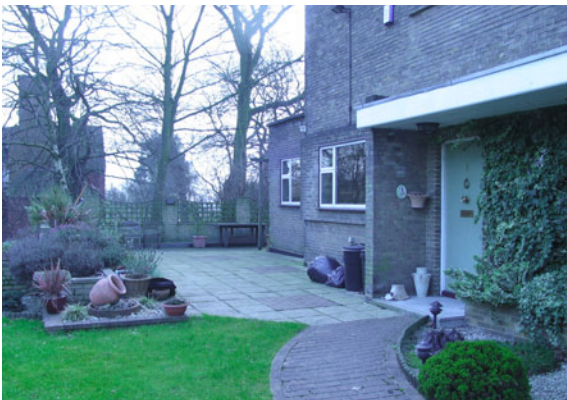
Poor quality hard landscaping materials, 2003
