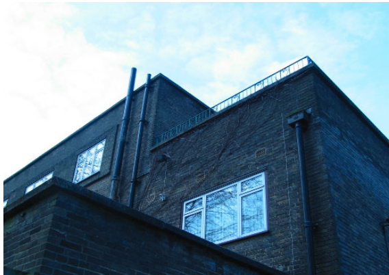
Rear elevation: flue and vines were removed
