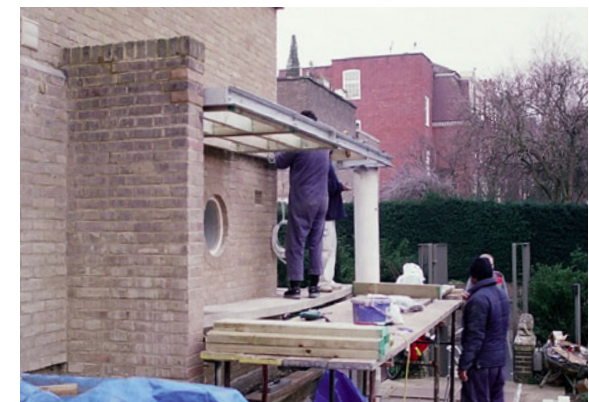
New steel framed canopy under construction
