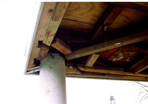
UPVC cladding removed exposing structure
