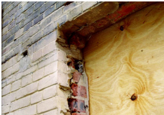
New opening showing facing brickwork and inner skin
