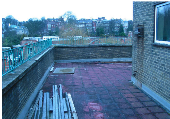
Existing 2nd floor terrace
