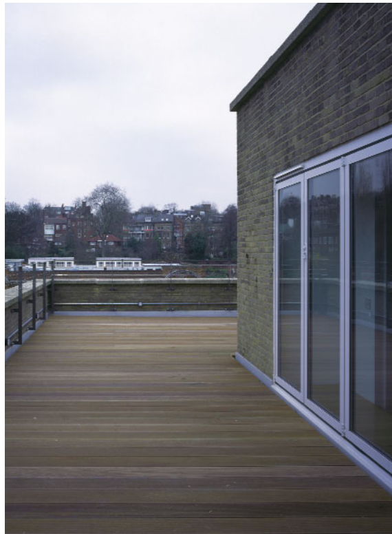
2nd floor terrace, new door opening and balustrade
