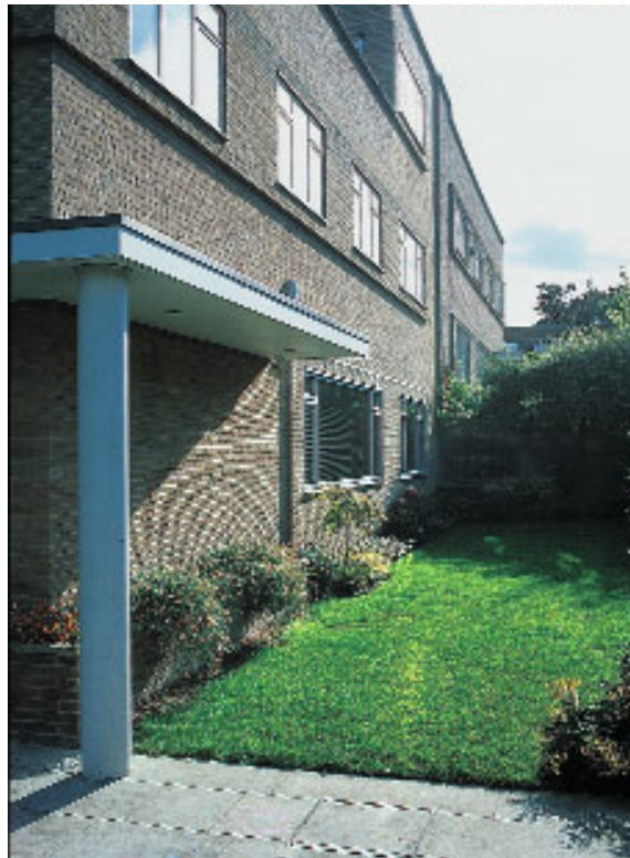
Reconstructed canopy and repointed brickwork
