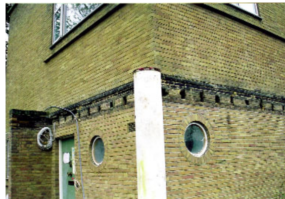
Existing canopy removed
