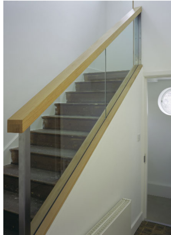
New stair balustrade
