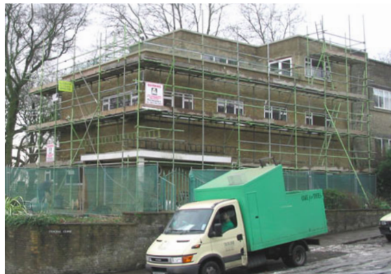
Brickwork cleaning and repair underway
